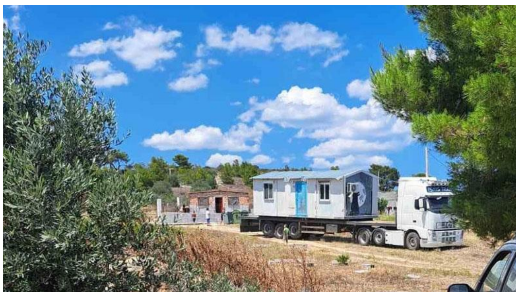
Prefabricated houses being moved by vehicles of the Municipality of Chalandri to the plot of land in the Municipality of Spata-Artemidon
